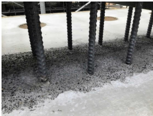
Figure 3: Roughness of concrete joint surfaces of horizontal joint area (No. 5)
