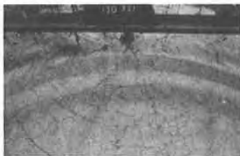
Figure 4. Crack Pattern in Dome at 130 psi (0.90 MPa)
