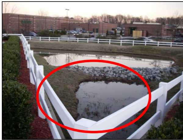
Figure 4.1. A wetpond with forebay circled.
