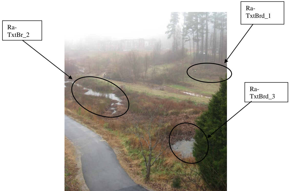
Figure M.3. Profile View of 3 Wetland Forebays on NCSU Campus
