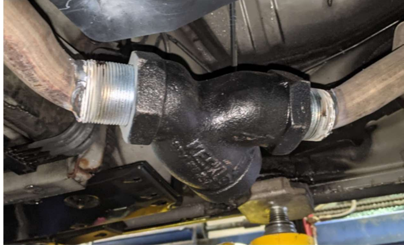
Figure 10. Cast iron wye joint in place.
