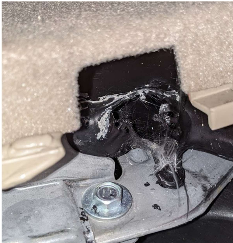
Figure 21. Damage to thermal management system inlet
