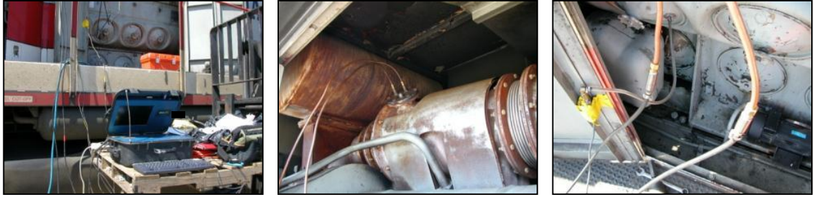
Figure 2-8: Installation of PEMS on a GP40 Locomotive Prime Mover Engine (a) PEMS main unit (front-view); (b) exhaust sampling port and metal tubes; (c) sensor array box
