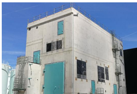
Figure 2. The EDF Diesel Ultime Secours (DUS) building
