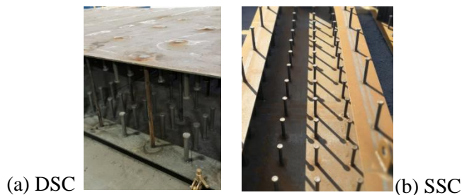
Figure 1. SC structural forms
