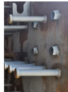
Nuts for bolting floor angle cleats
