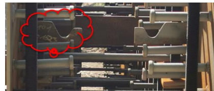
Support bracket for dowel bar
