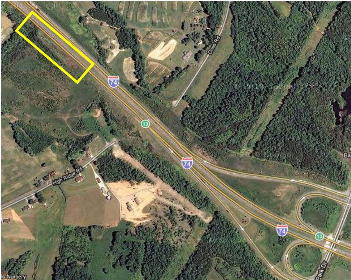
Figure 3.3 Aerial imagery of Mount Airy research site (Google Maps, 2011).
