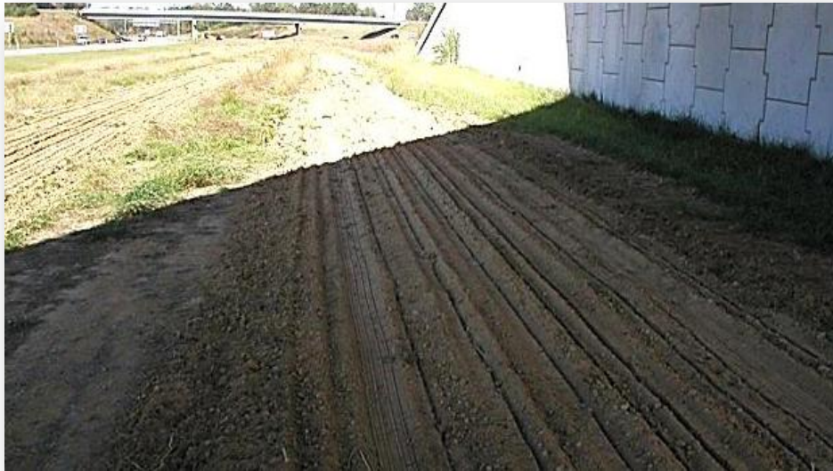
Figure A2.1.5 Seedbed following maximum tillage and planting at Knightdale research site (photo courtesy of NCDOT).
