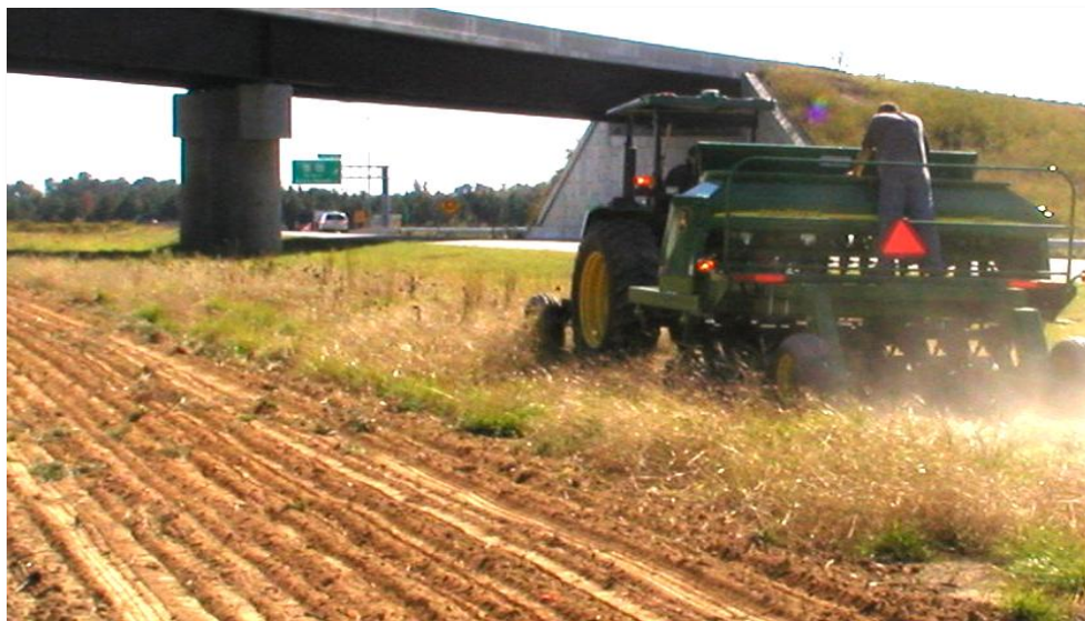
Figure A2.1.4 Seedbed preparation by minimum tillage treatment (left) and no-till planting (right) at Knightdale research site (photo courtesy of NCDOT).
