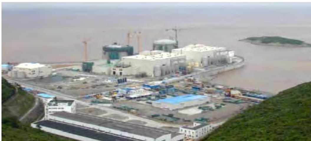
Figure 10 Qinshan Phase 3 CANDU Power Plant
