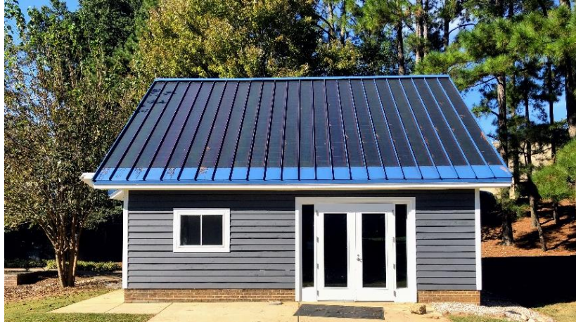
Figure 1.4: The garage PV system.
