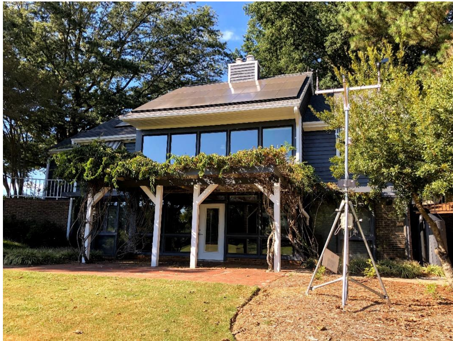
Figure 1.1: The house PV system.
