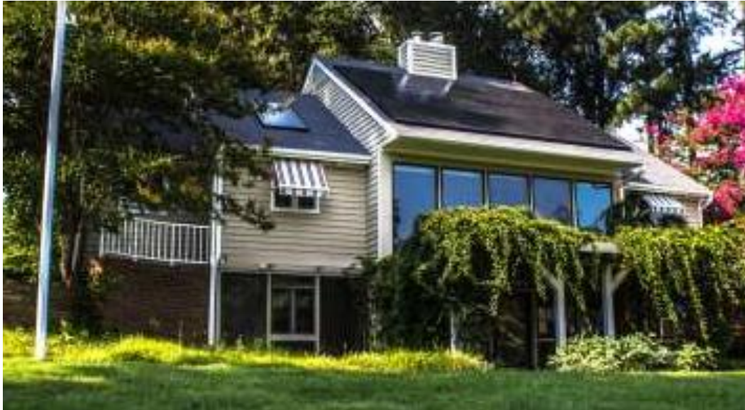
Figure 5.6: Shading from a tree on the western side of the Solar House.
