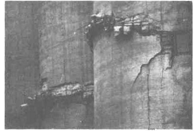
Fig. 7. IV) Direct and indirect effects of lack of transversal reinforcement in bidimensional structural elements.
