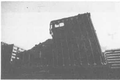
Fig. 8. IV) Greater ductility (e. g. achievable by making use of spirally reinforced columns) can have a harmful effect if attained at stiffness expense because it involves a greater demanded ductility.
