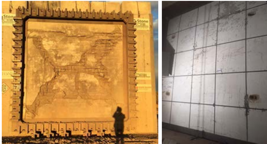
Figure 2. Front and rear face of the slab after Test 1
