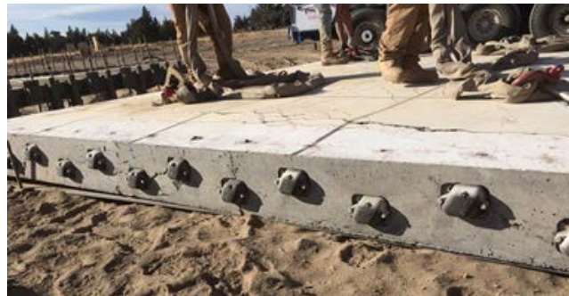
Figure 9. Through-thickness crack at the cable anchors and a crack along the edge at one slab thickness from the edge in Test 3
