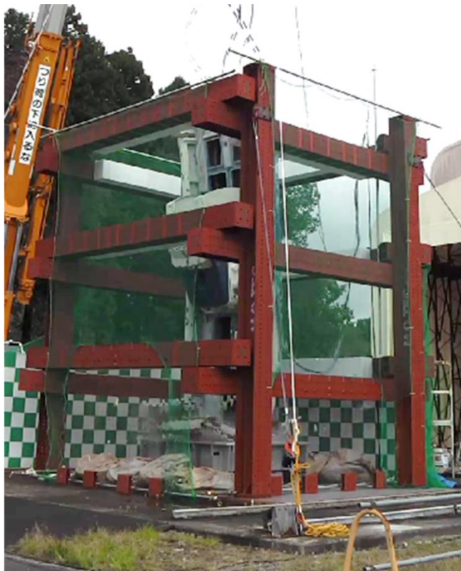
(a) Situation immediately after the collision experiment
