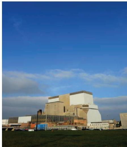
(Courtesy of EDF Energy)
