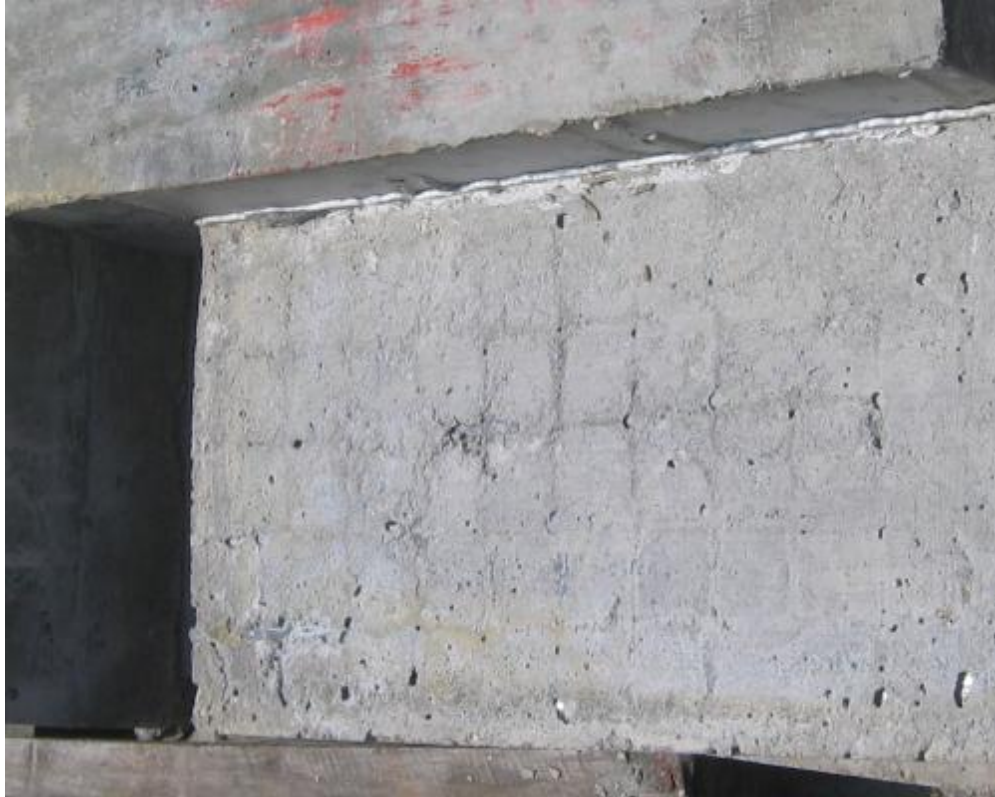
Figure 4-12 Specimen B3 interface (premature debonding failure)
