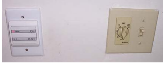
Figure 5.2.3: Dimming Switch and Louver Timer
