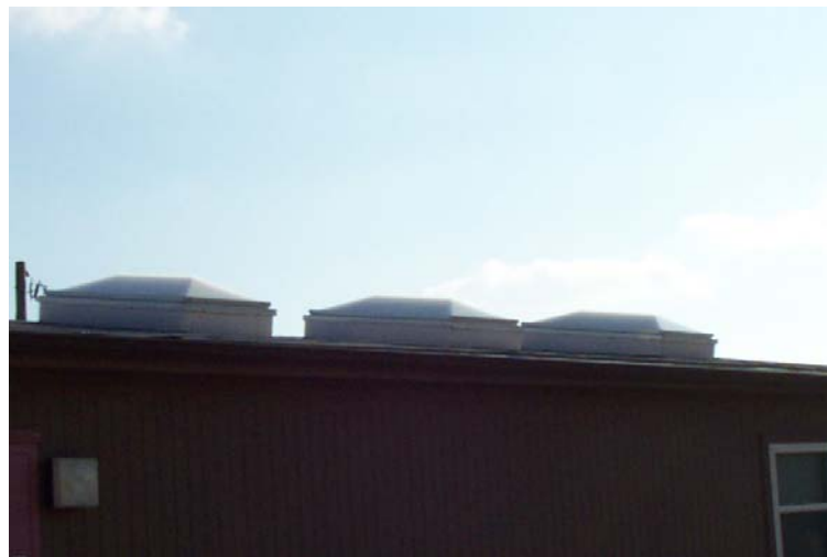
Figure 5.4.1: Outdoor View of Skylights
