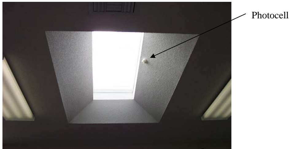
Figure 5.2.2: Skylight View and Photocell Location
