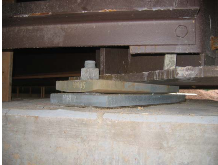
Figure 3-15 Pot Bearing of Wilmington Street Bridge
