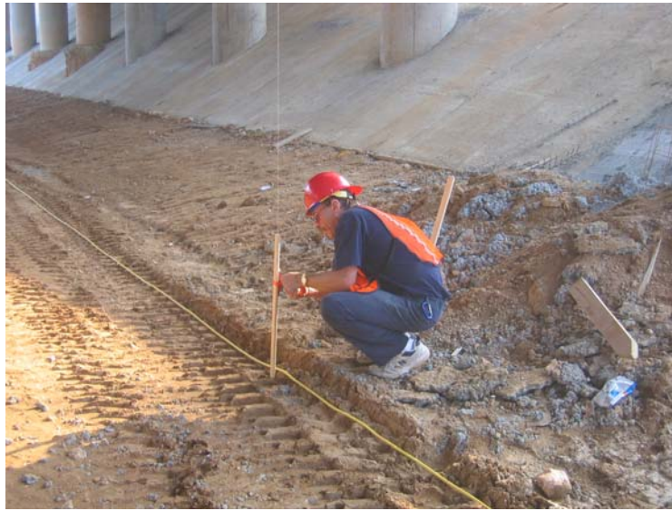
a) Wooden Stake Installation
