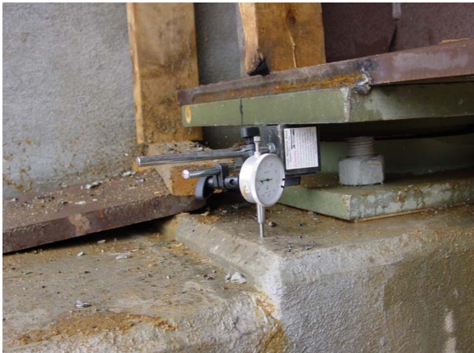
Figure 3-12 Dial Gage Placed at End Support of Girder
