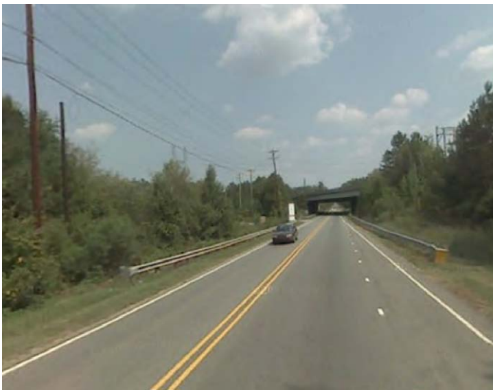
FIGURE A-2. Underpass Downstream of ATL Merge (40)
