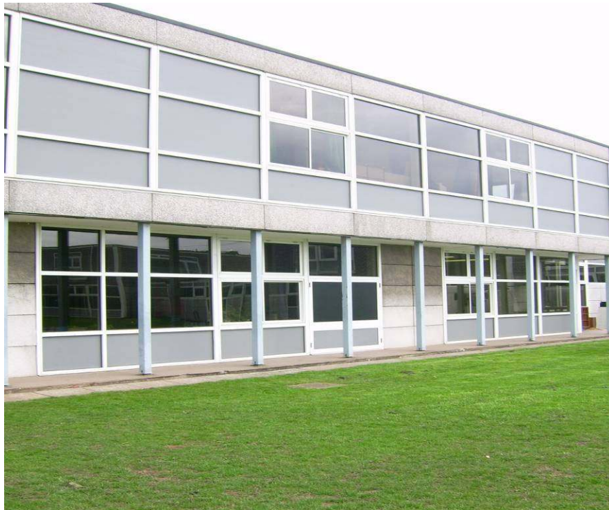
Figure 2.4 Architectural Sandwich Panels
