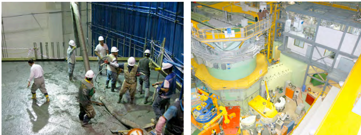
Figure 2. Placing of heavyweight concrete and completed shielding room in reactor hall
