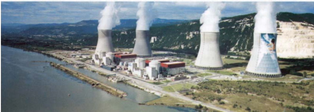
Fig 1: the four PWR units of Cruas, France, provided with seismic isolation.
