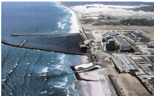
Fig 2: the two PWR units of Koeberg, South Africa, provided with a seismic isolation system composed by rubber bearings coupled with friction plates.
