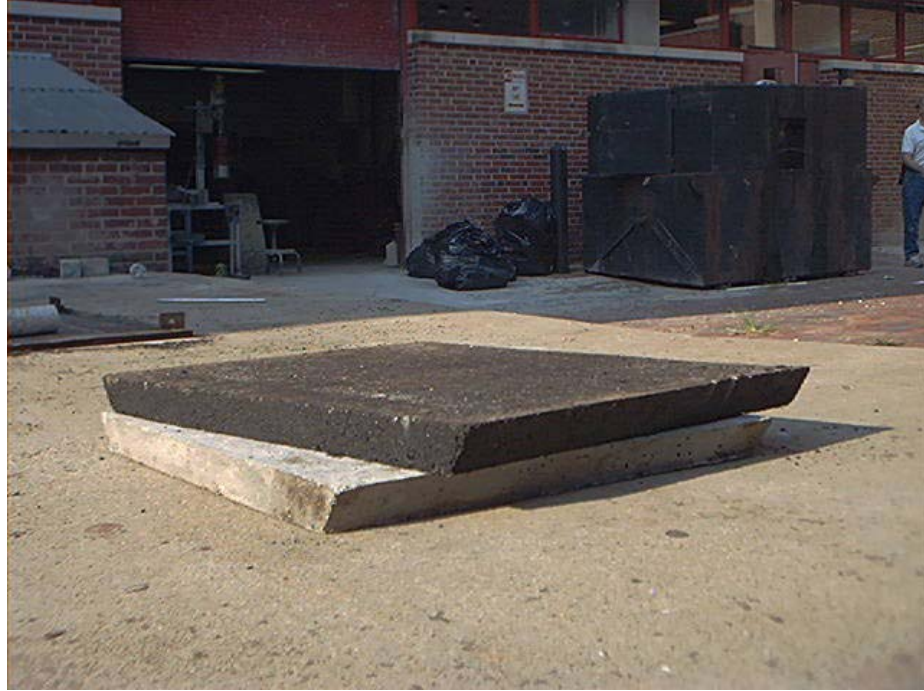
Figure 8-15 Debonding of composite PCC-AC specimen without tack coat
