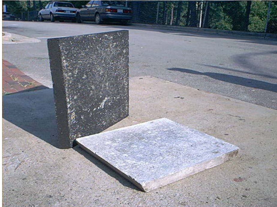
Figure 8-16 Debonded composite PCC-AC slabs without tack coat
