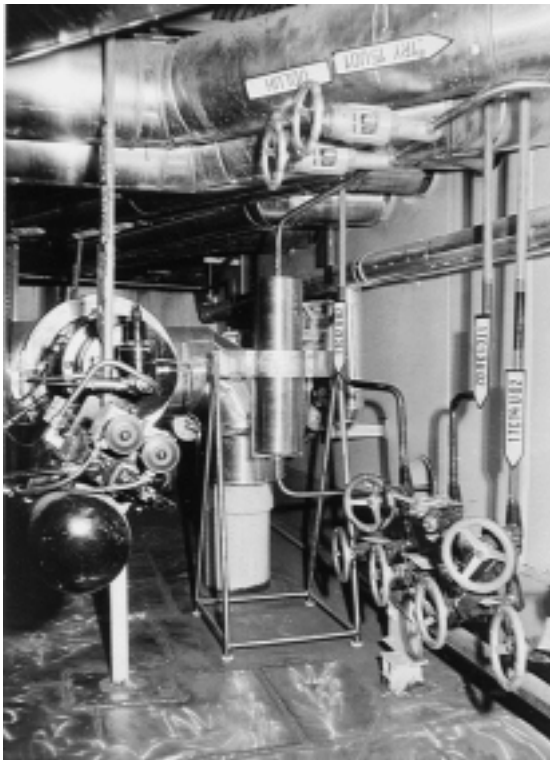
Fig. 1 Global view on the corrosion chamber
