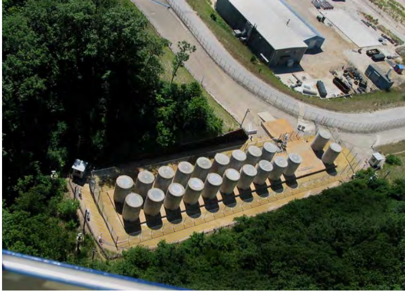
Figure 1: Typical Vertical DCSS on Pad at a Nuclear Power Plant
