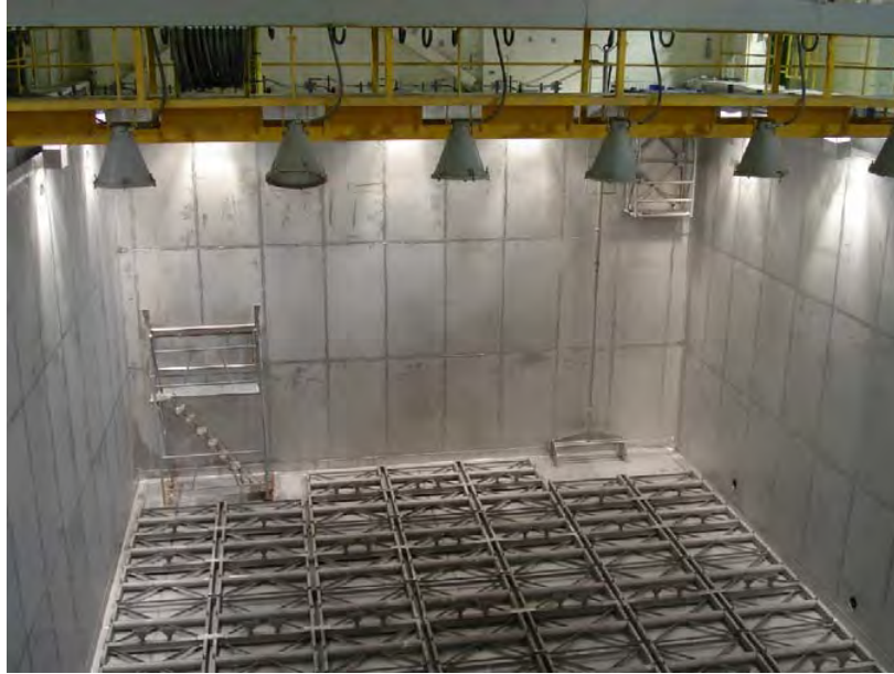
Figure 4 - Spent Fuel Storage Bay Liner after the Pickling and Passivation
