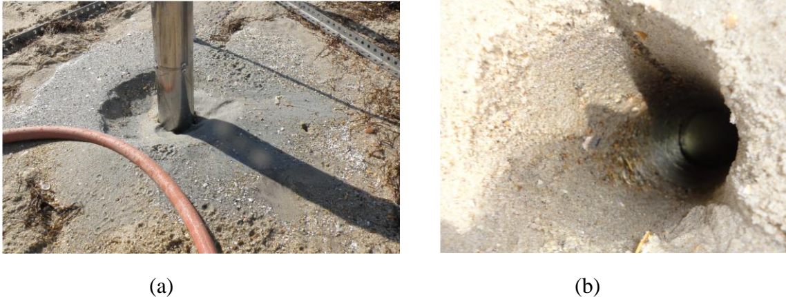
Figure 6. Depth Test Scour Profile (a) at t = 10 sec and (b) After the Test.
