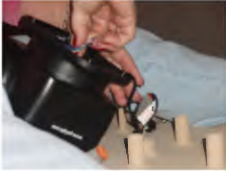
Step 8: Wire and secure Go-Light on roof on mounting bracket
