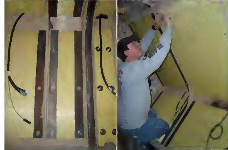
Step 8: Grind off stud ends flush with nut using angle grinder
