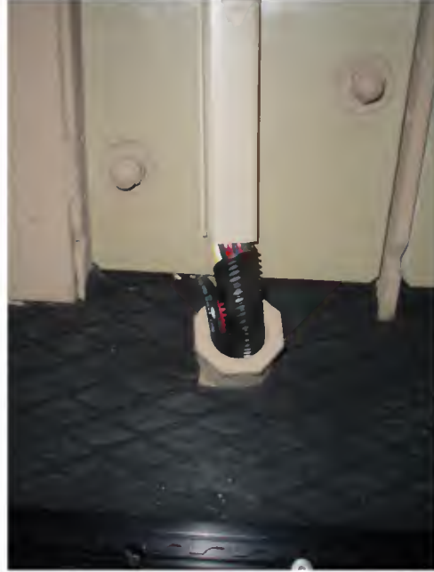
Steps 2-4: Insert wires into raceway and attach to wall
