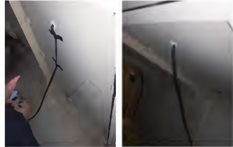
Step 6: Grab 4 interior wires, route and secure with Velcro
