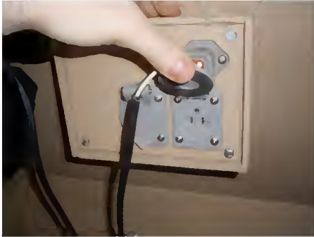
Step 6: Check 120V outlets
