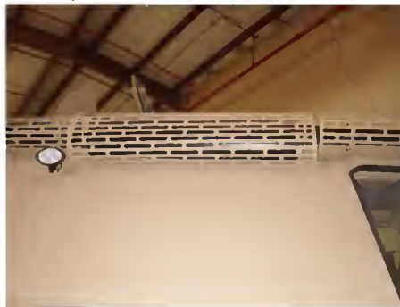
Steps 8-9: Obtain and secure exhaust cover shields
