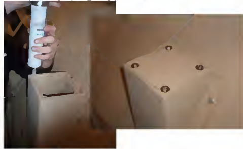
Step 6: Bolt down cover plate Step 7: Repeat for other antenna boxes
