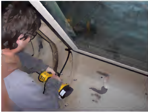
Step 4: Chase wall blocks to remove paint from threads
