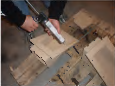
Step 2: Run a bead of silicone caulk around antenna box edge
