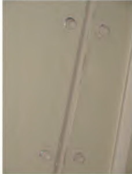
Step 2: Tighten acorn nut on end of each exposed Goldshield stud.
