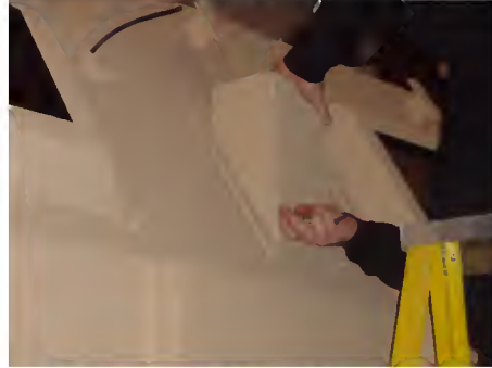
Step 5: Run silicone caulk around antenna box cover edge
