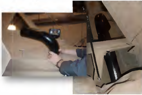
Steps 3-4: Align and secure 90° pipe through front into engine
