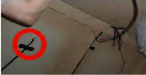
Step 4: Route wires through inner wall and attach with Velcro
