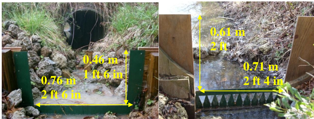
Figure 5. From left: inflow and outflow weirs.
