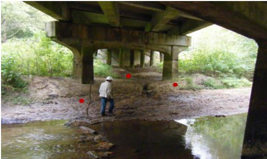
Figure 8.1 Example of low-head space required for drilling from the bridge deck (top of bridge).
