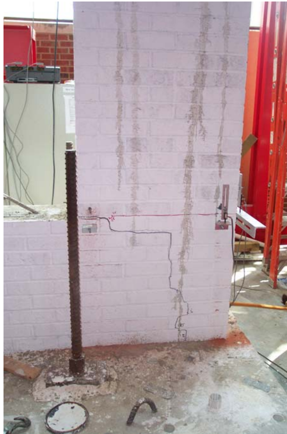
Figure 12: Initial Crack in Wall 2
