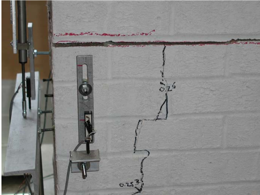
Figure 3: Base Crack at 0.75 Drift Ratio
