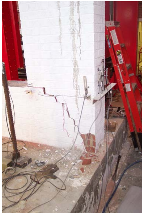
Figure 8: Continued Vertical Crack Growth Resulting Entire Side of Wall Rocking at 1.75 Drift Ratio
