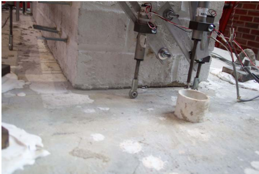
Figure 14: Masonry Wall "Damage" After 56 Earthquake Runs
