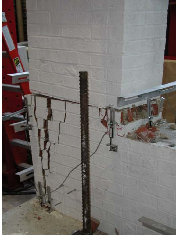
Figure 6: Crushing of Masonry at 2.25 Drift Ratio
