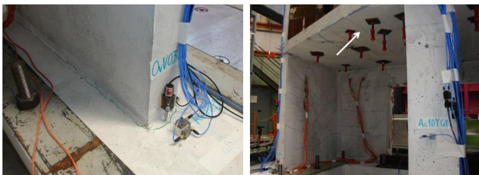
Figure 6. Crack at the bottom of wall 04 after Northridge 0.40 g (left); final state of SMART2013 (right), Richard et al. (2018)
