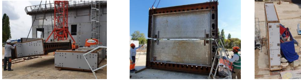
Figure 20. Pool floor modules assembly and butt welding on the ground
