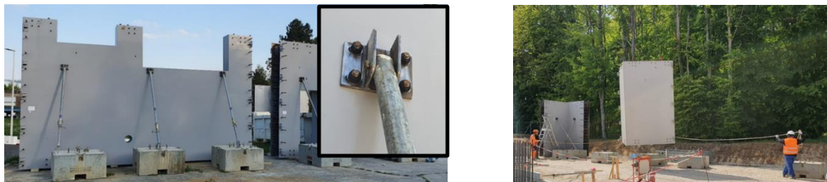
Figure 4. Wall modules storage with stabilizing props (left) - wall module transfer (right)
