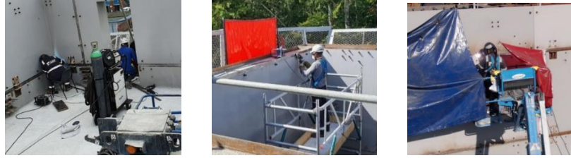
Figure 14. Fillet welding (left) - plate grinding (middle) – APC shell butt welding (right).
