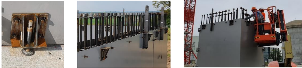
Figure 5. Levelling jack (left) – vertical guides (middle) – dowel bars raising (right)
