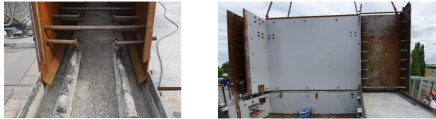
Figure 11. Level 5 module with backing plate (left) - APC shell module installation (right)
