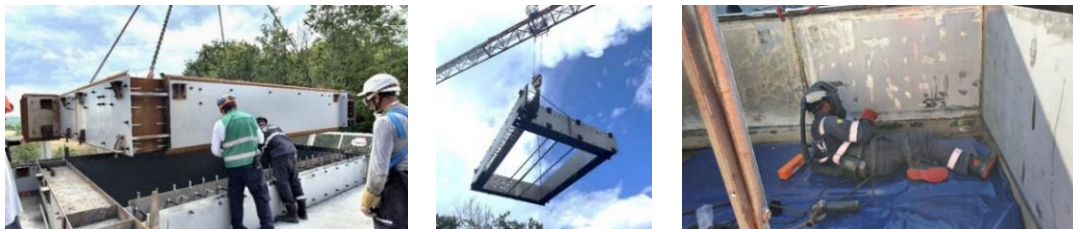
Figure 22. Pool modules installation (left and middle) – horizontal joint butt welding (right)
