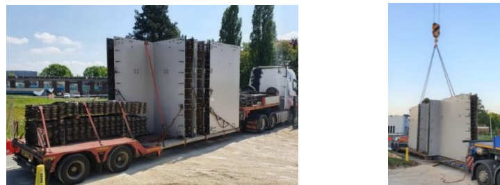
Figure 3. Wall modules stored on a truck (left) - wall module unloading (right)
