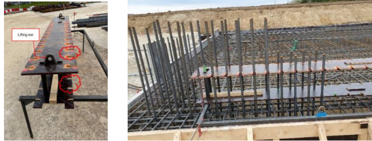
Figure 2. Template tool (left) - starter bars installation in the template tool (right)
