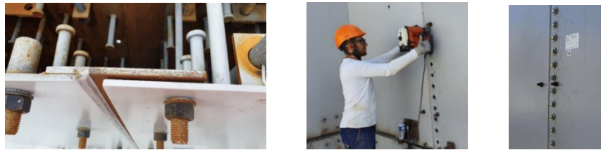
Figure 15. Pre-stressed bolted connection – joint with straight backing plate before holes drilling (left)
