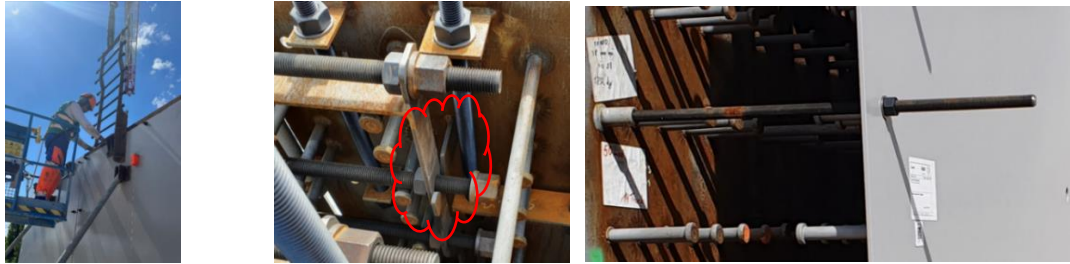
Figure 8. Horizontal dowel bars installation (left) - frame bracket (middle) - removable tie-bars (left)
