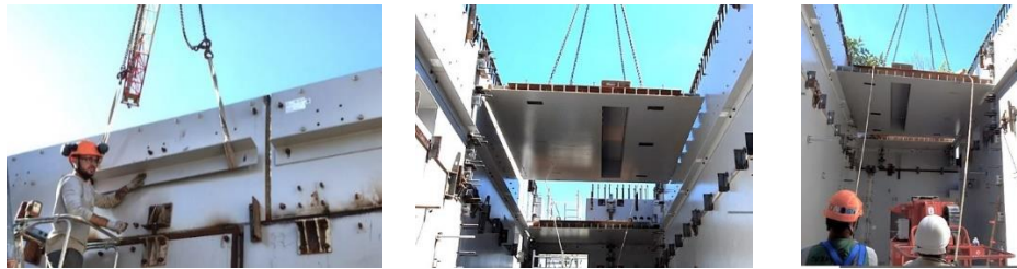
Figure 17. Support L angle installation (left) - floor module installation (middle and right)
