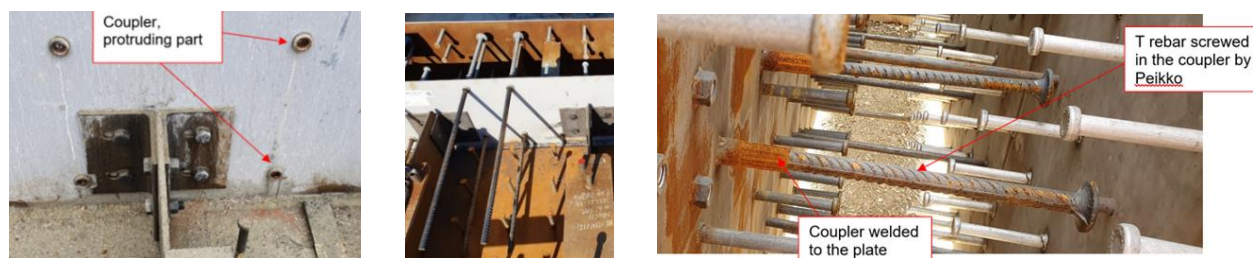
Figure 19. Slab rebars anchorage in the wall modules
