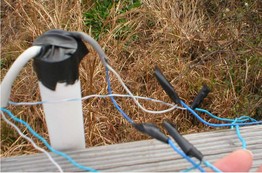
Figure 1.7. Showing wires from multiplexer to PVC pipe and electrical tape.
