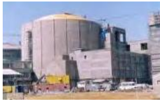
(b) Completed Containment
