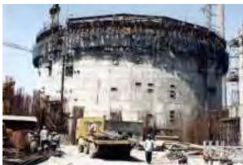
(a) IC under Construction
