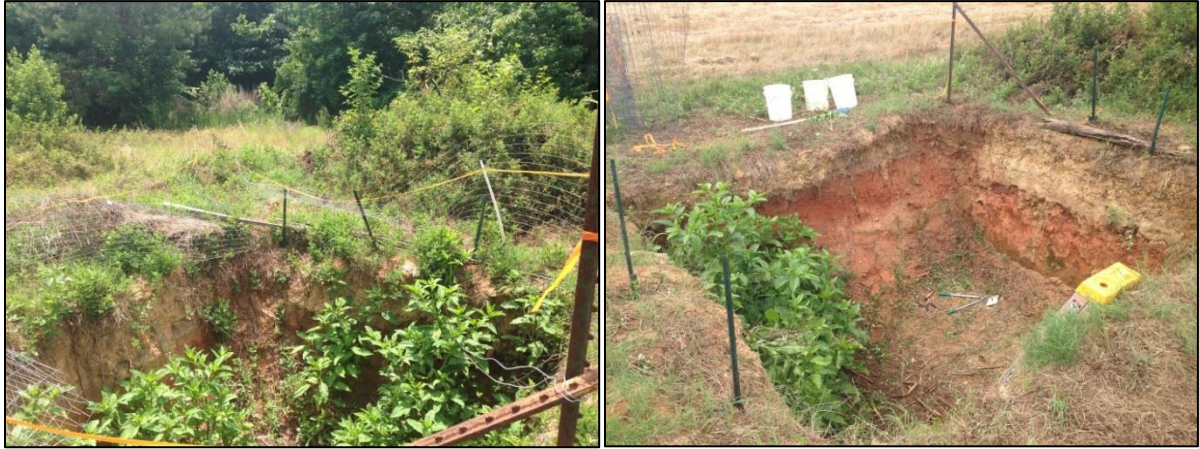
Figure 3.1: The Lake Wheeler Field Site Being Renovated
