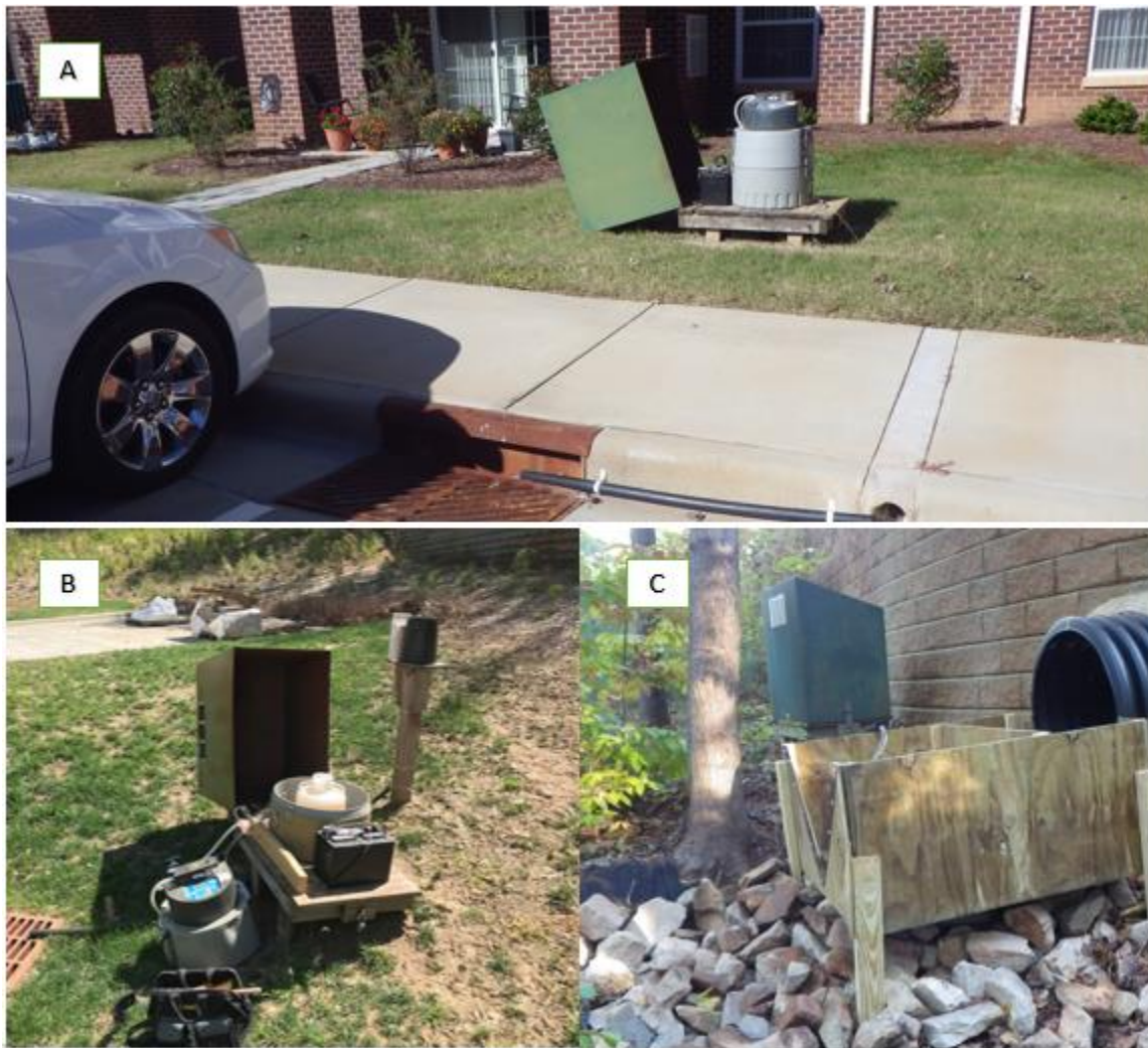
Figure 2-6. Monitoring Stations at Capital Oaks: (A) Station “Park” monitors roof and parking lot runoff from the western portion of the watershed (B) Station “East” monitors roof, parking lot, and unpaved/grassed runoff from the easter portion of the watershed parking lot (C) Station “Out” monitors effluent leaving the outlet structure.
