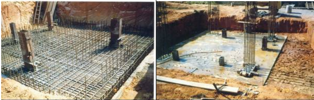
Fig.3 Construction of Raft Foundation with Rock Anchors
