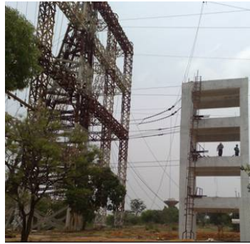
Fig.4 (a) Structure at Tower Testing Facility
