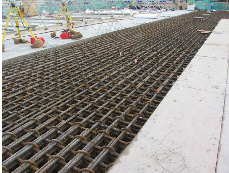
Figure 7. Slab reinforcement
