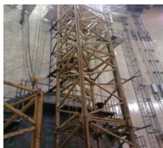
(b) installment of the structure
