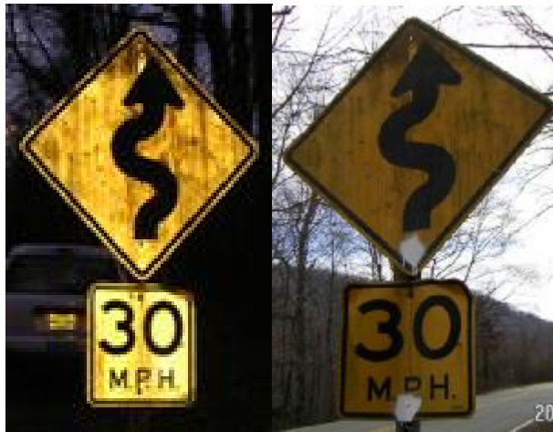
Figure 7.14. Sign Damaged Due to Tree Sap
