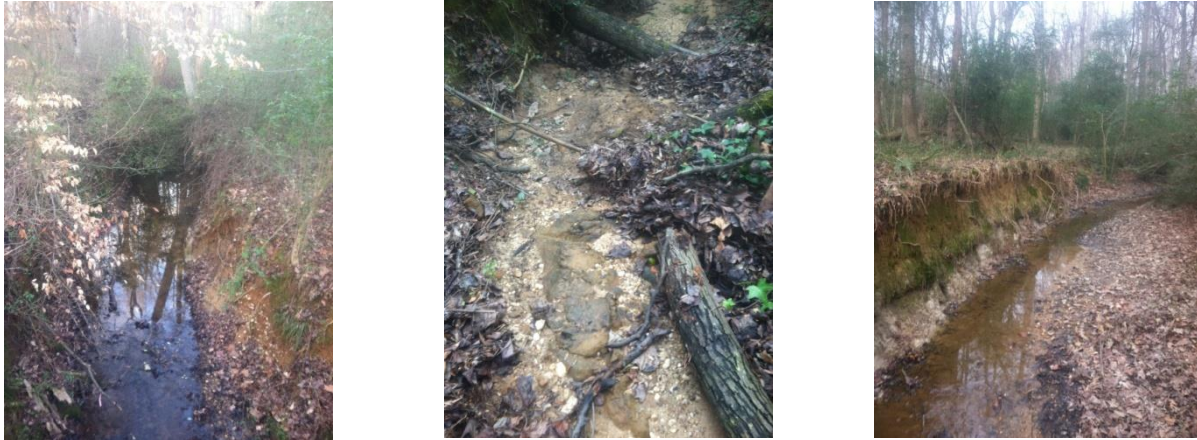
Figure 4: Stream Channel substrate change, Erosion and Narrowing.
