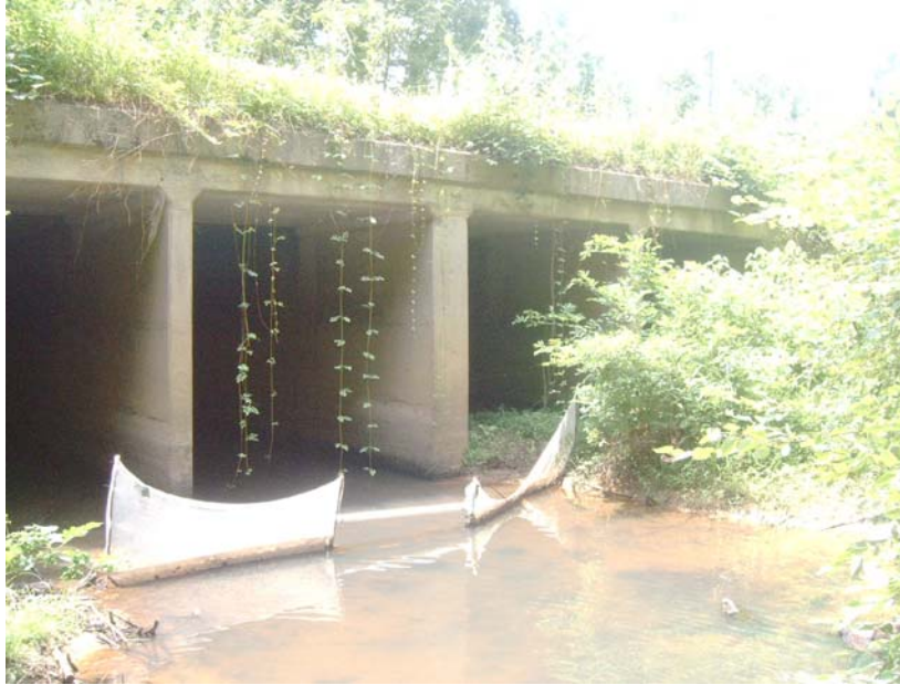
Figure 4. Bankfull Bench Forming in Culvert.
